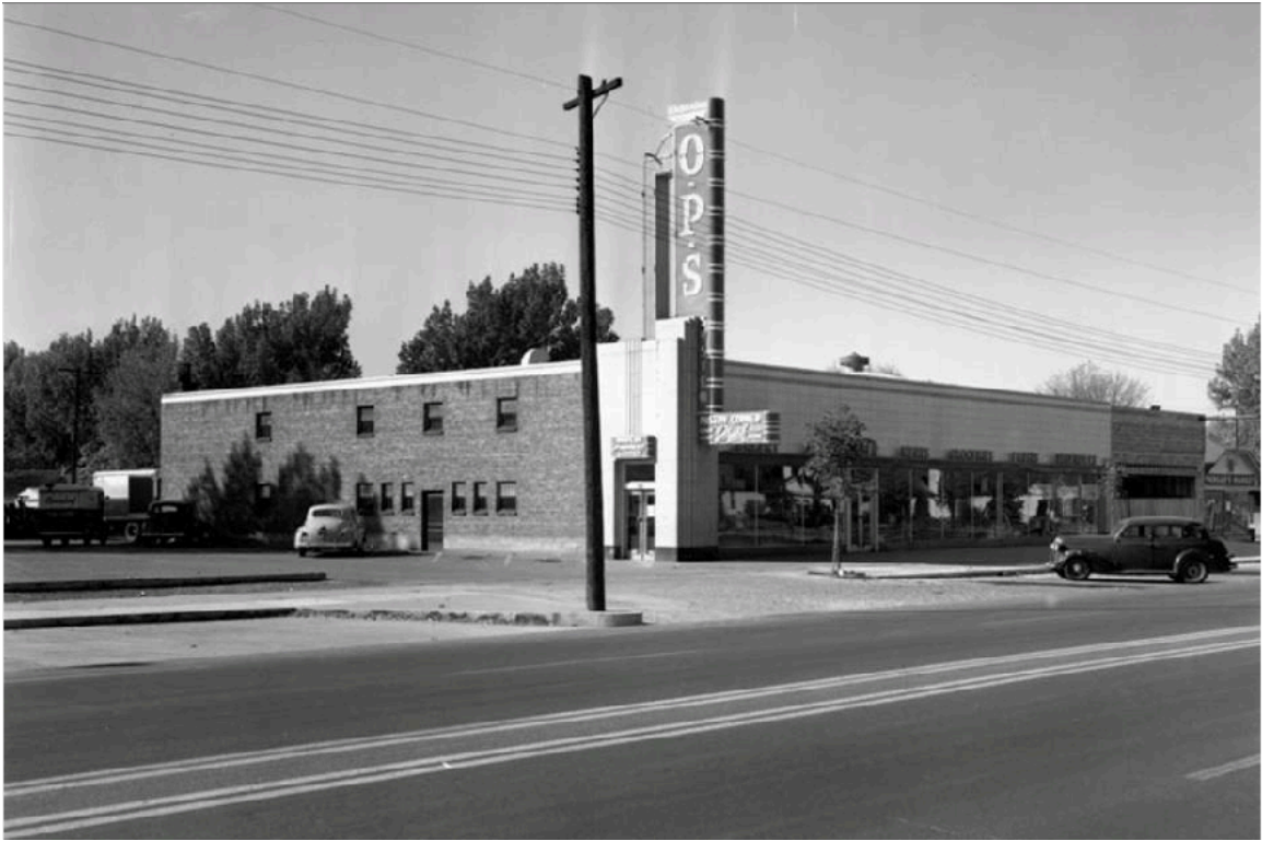
Historic Photo - Original Facade - O.P. Skaggs - Northeast View
